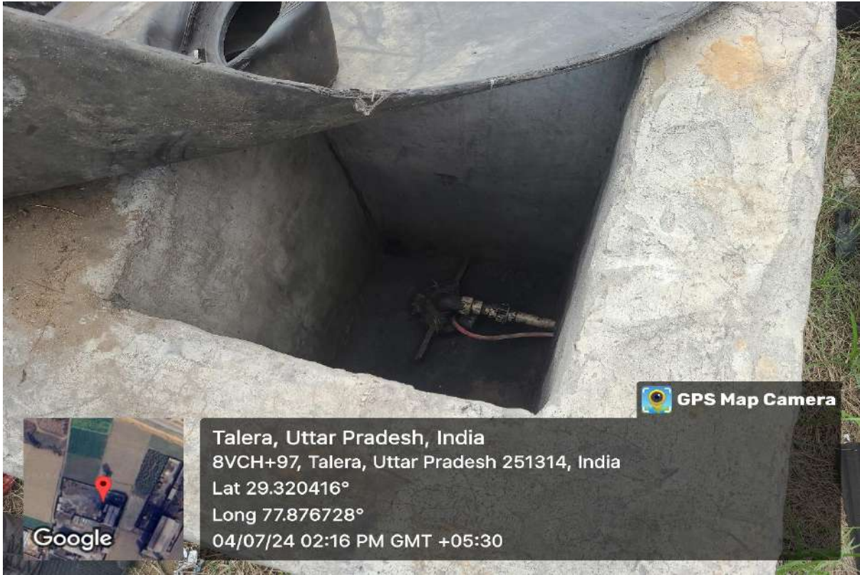
Figure 10 Borewell inside unit's premises
