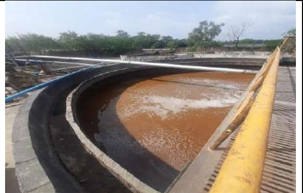
Treated effluent before recycling to process
