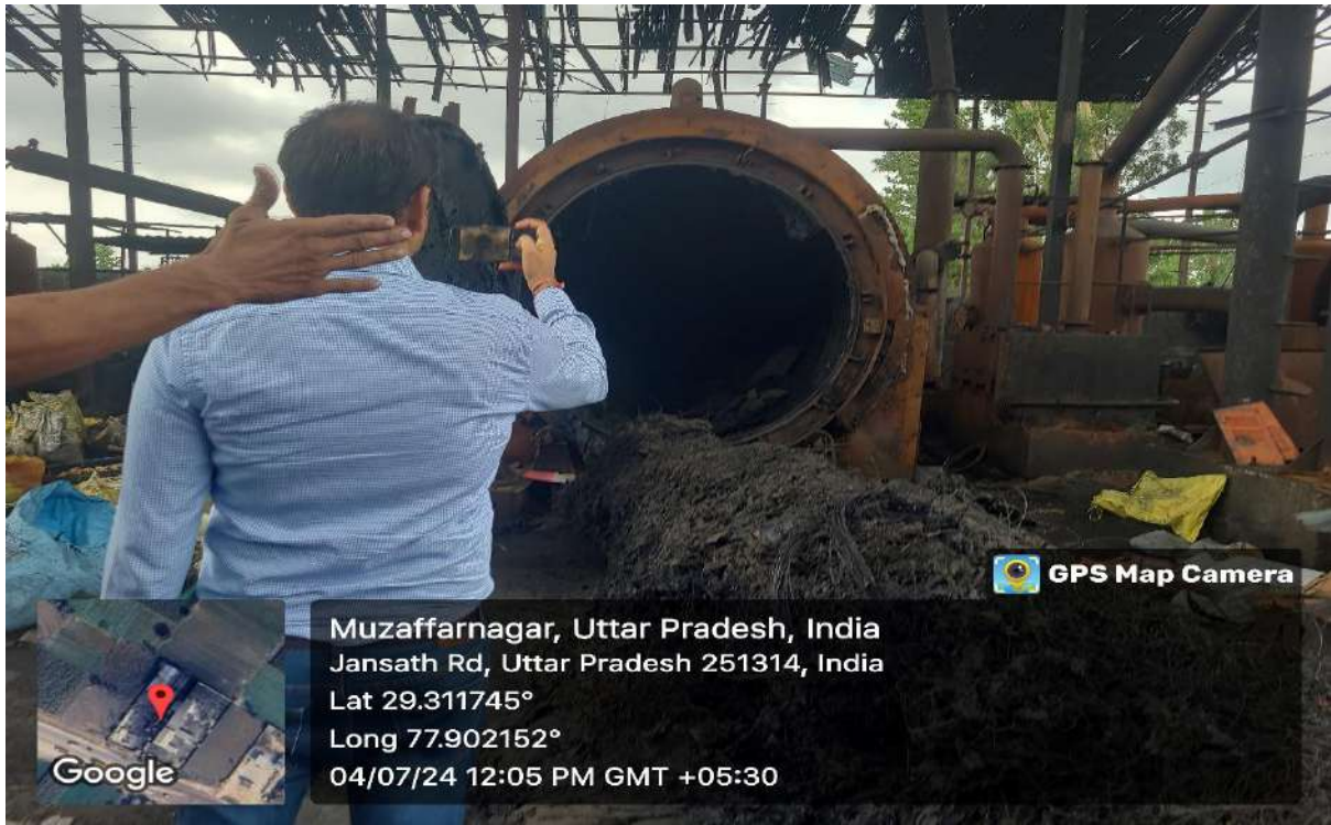
Figure 3 Pyro chamber cleaning
