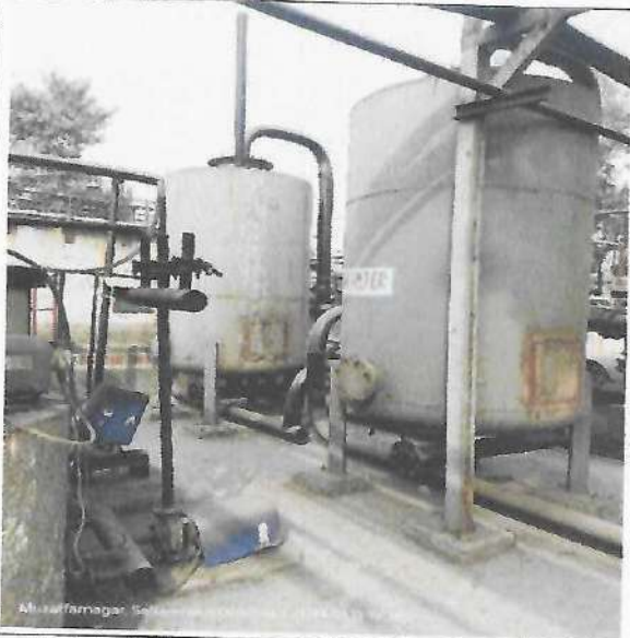
Fig.10: APC system and Stack attached to Boiler
