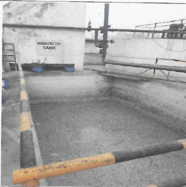
Equalization Tank
