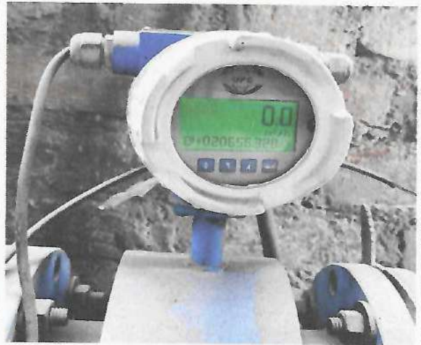
Flowmeter reading of Borewell No. 2
