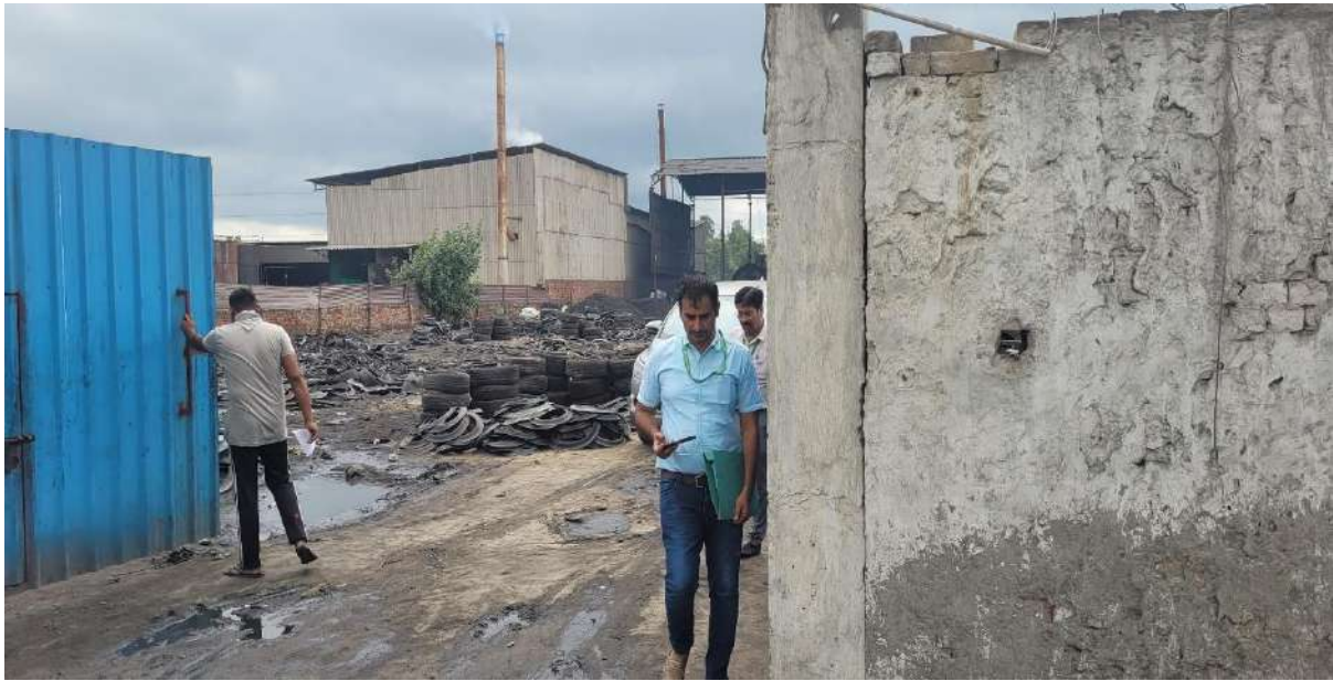
Figure 1 Main entrance gate of the Unit
