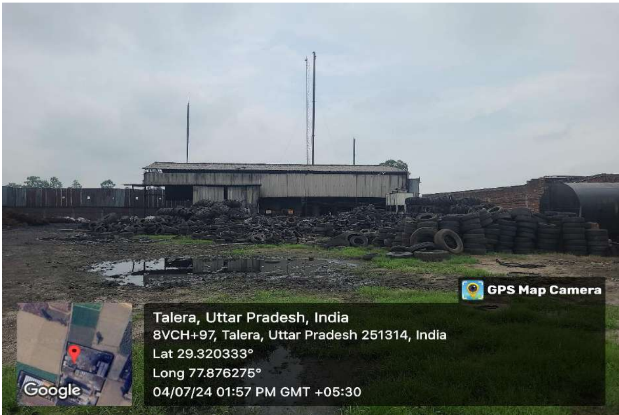
Figure 2 Unit premises and stored tyres inside premises
