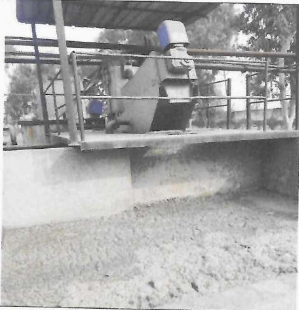
Fig.9: Mechanical system for sludge dewatering
