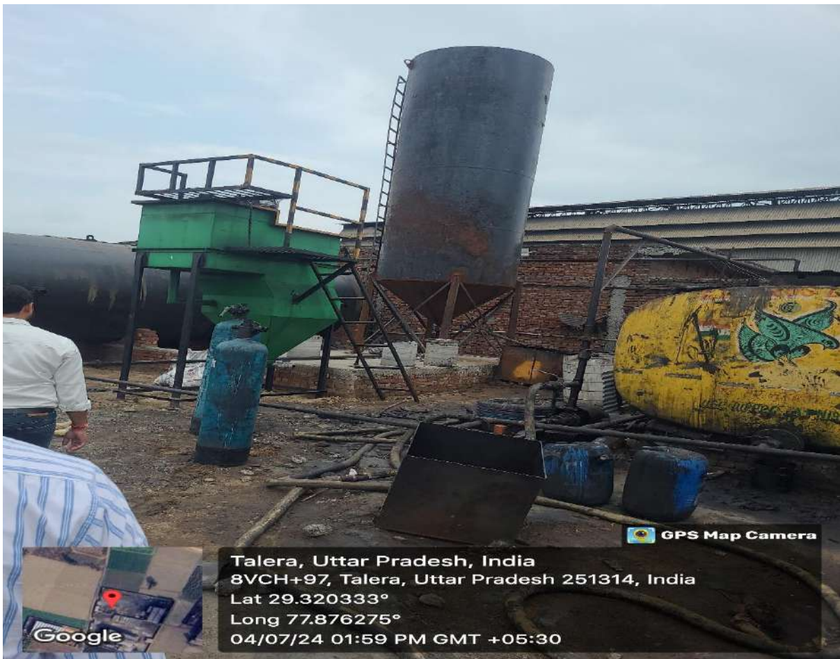
Figure 3 ETP system yet to be installed
