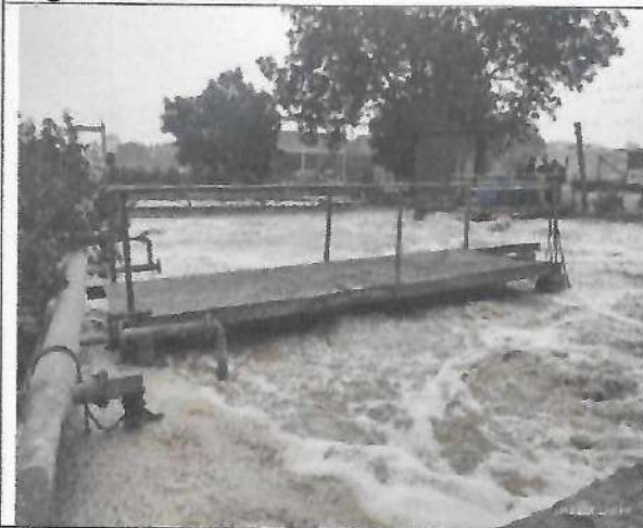
Fig.5: Aeration tank
