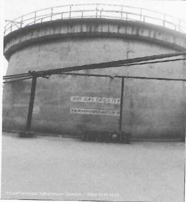
Fig.4: Bio-digester (Anaerobic Treatment)
