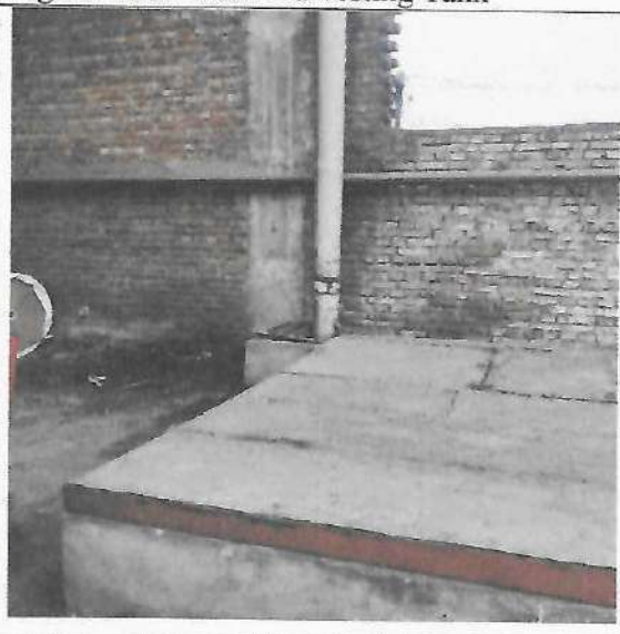
Fig.16: Rain Water Harvesting Tank
