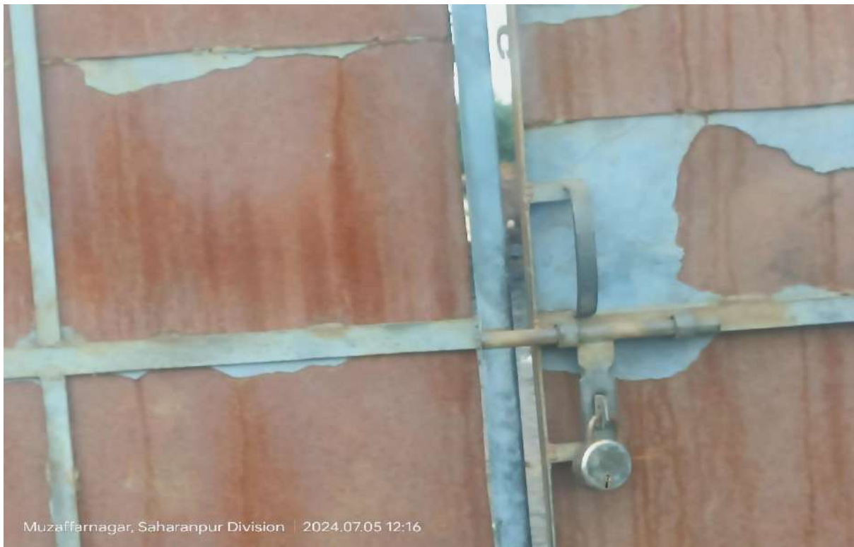
Figure 2 Lock at main entrance gate
