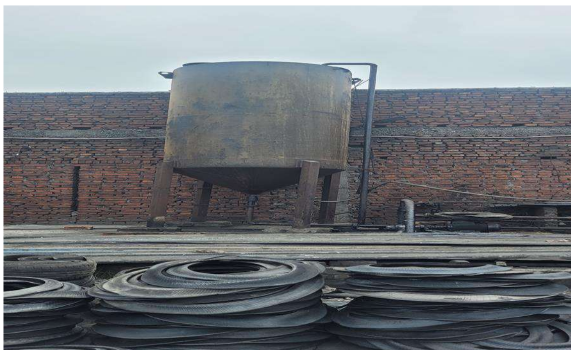
Figure 6 Pyro Oil storage and filter
