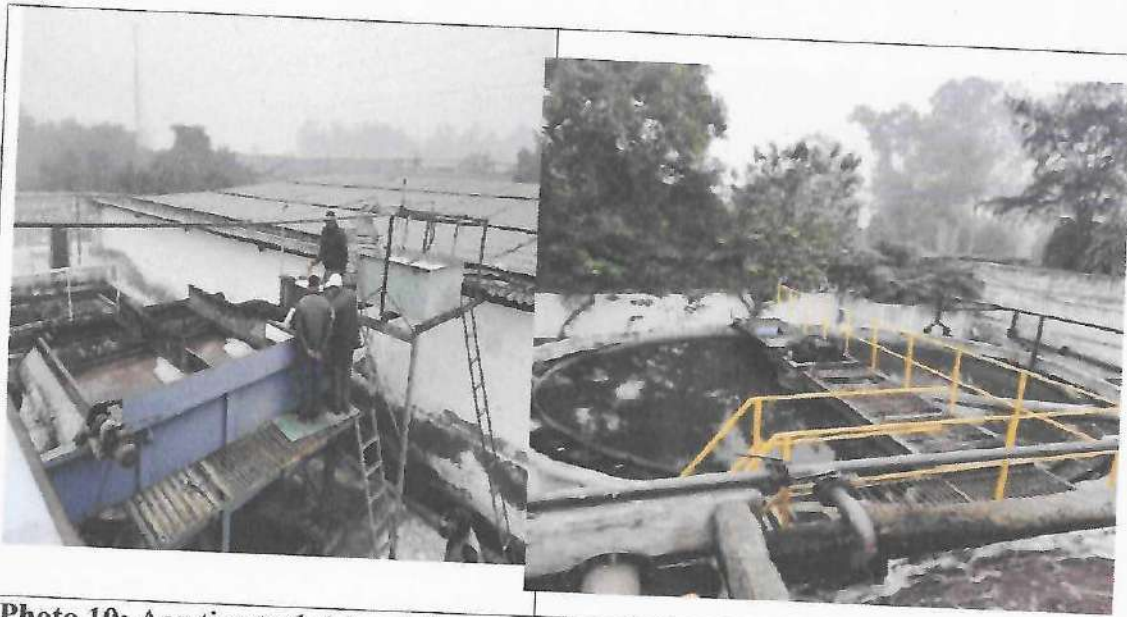
Photo 10: Aeration tank (s) and Sec. clarifier
