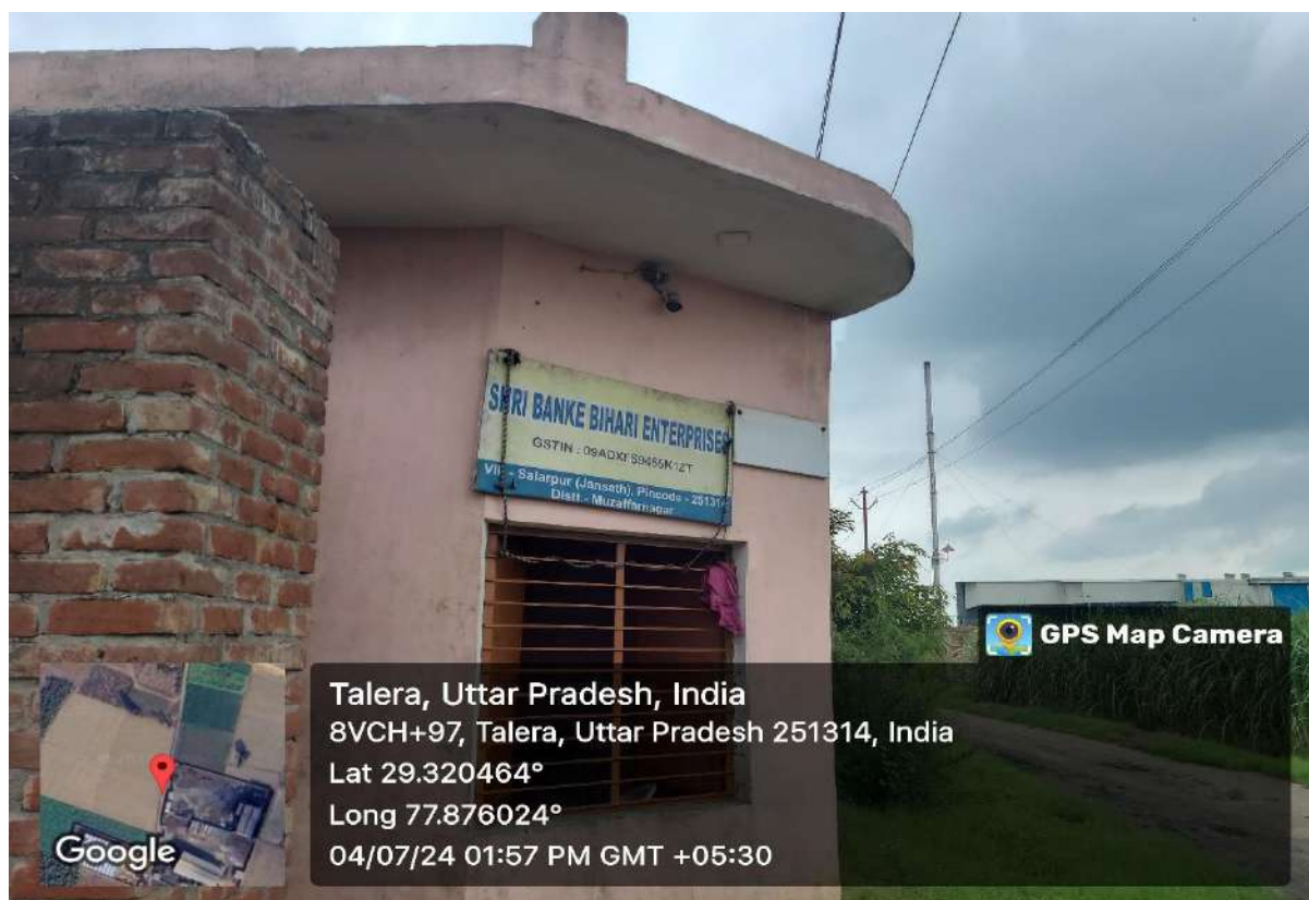
Figure 1 Main Entrance gate of the Unit
