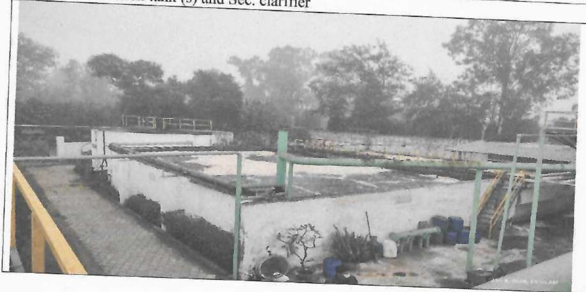
Photo 10: Aeration tank (s) and Sec. clarifier
