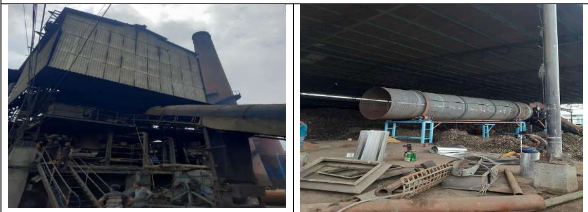
Modification of existing boiler to RDF based boiler
